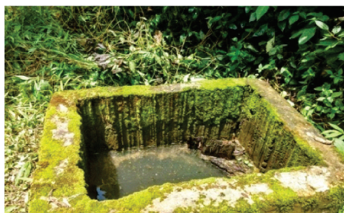
Figure 1: Concrete salt well
